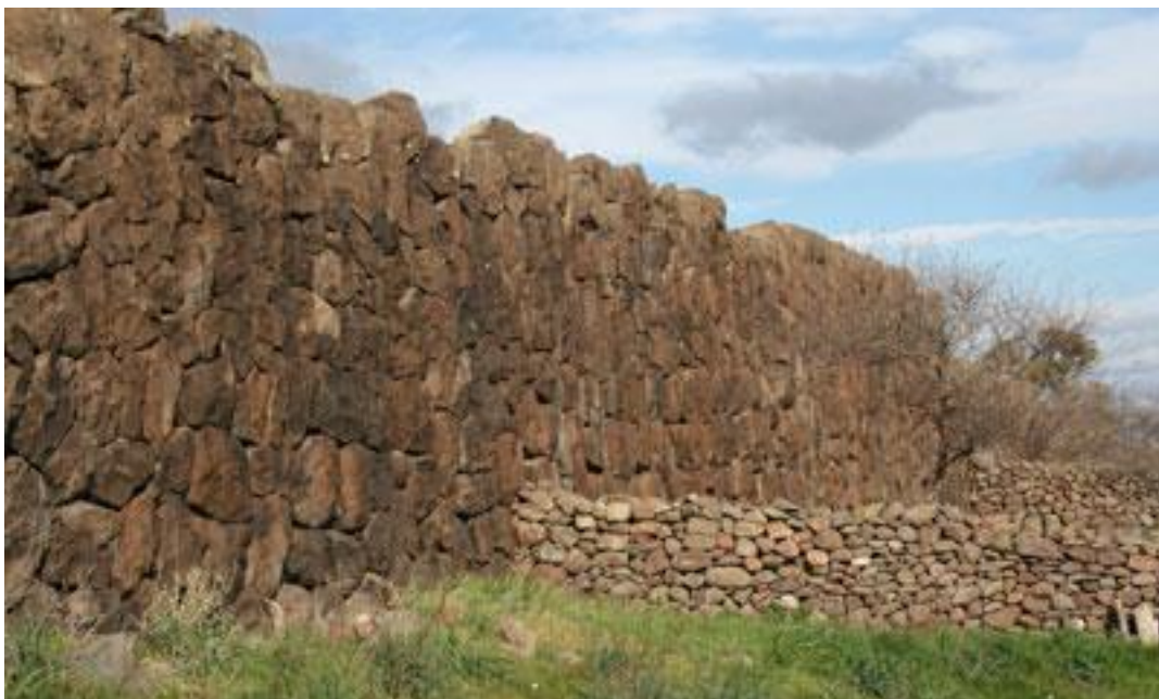
The well-built ("kaloktistos") retaining wall
