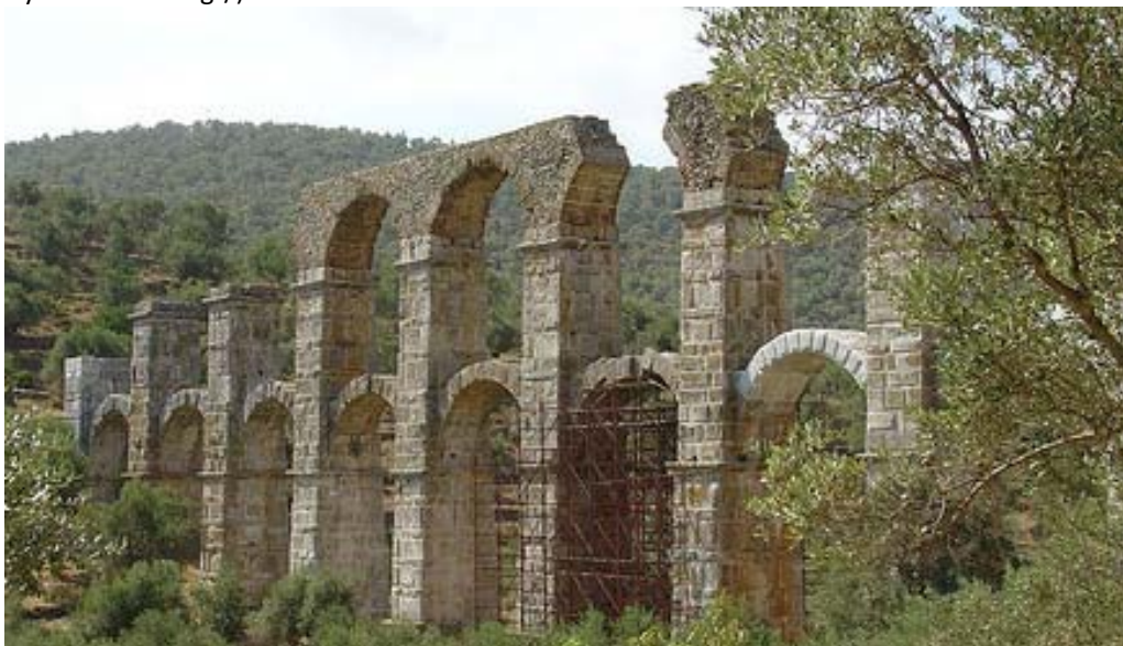
The Roman aqueduct at Moria
